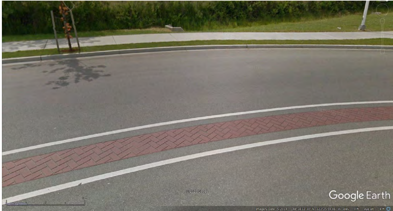
Figure 15. Photograph. Lane divider for turbo roundabout at Victoria International Airport. (31)
